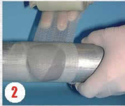
2 Apply RAPP-IT BANDAGE over the Steel Putty.
