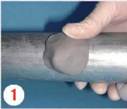
1 Apply RAPP-IT STEEL PUTTY to leak site and mould.
